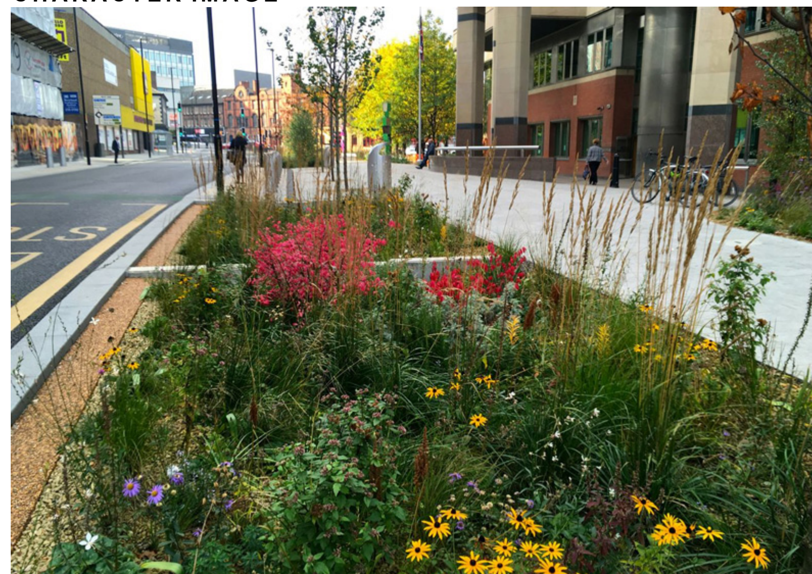
1. Widened boulevard with raingarden separating sidewalk and roadway
